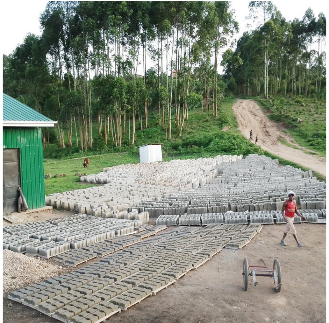
Zero-cement precast blocks and pavers made with new binders on site in Rubanda. The materials produced will be used in developing a climate resilient and functional rural homestead for a member of the local community
