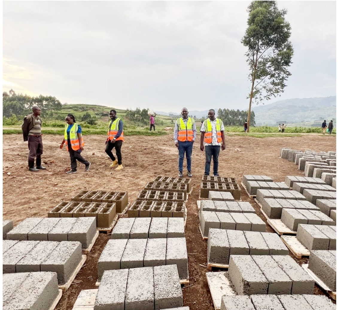
Concrete blocks produced out of zero-cement binders being piloted on site in Rubanda
