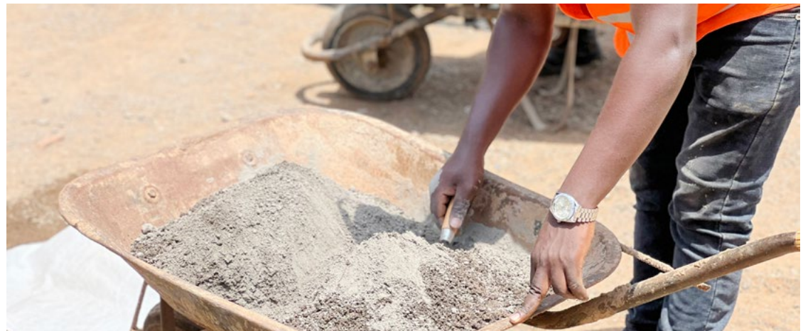
Alternative binders trial mixes on site
